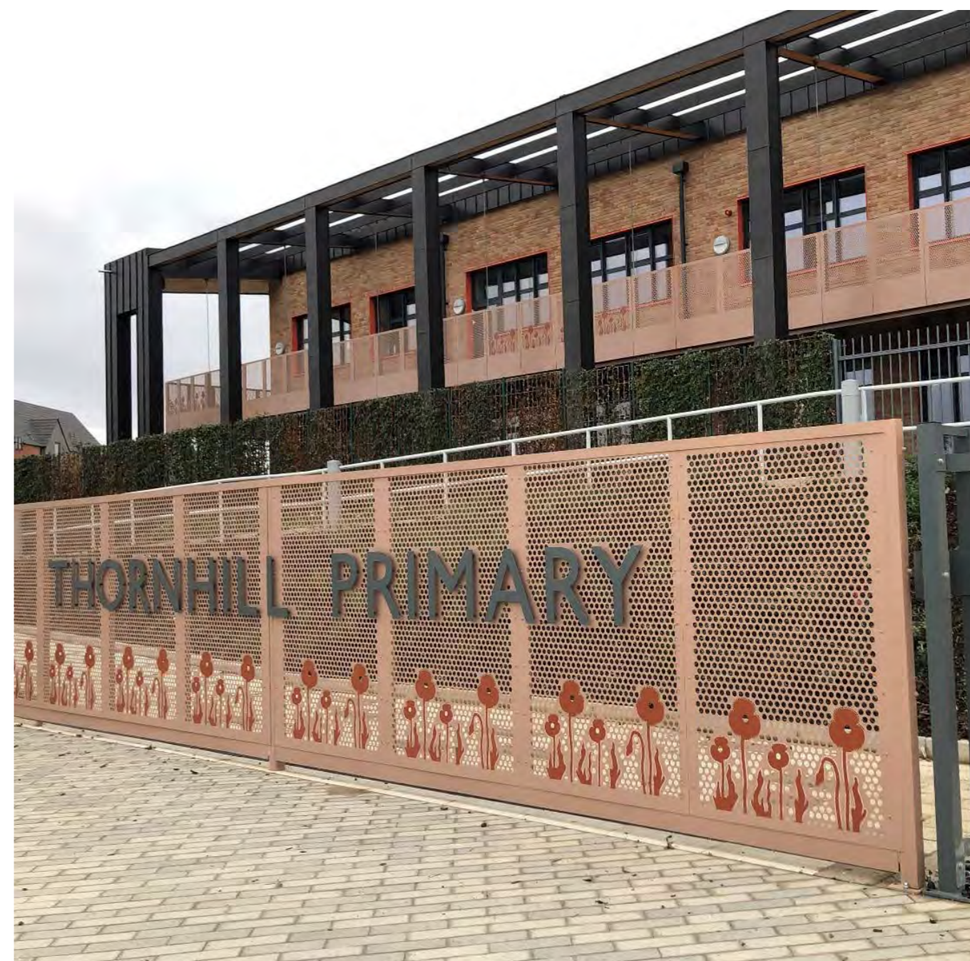
Figure 285: Thornhill Primary School, built to Passivhaus standards
