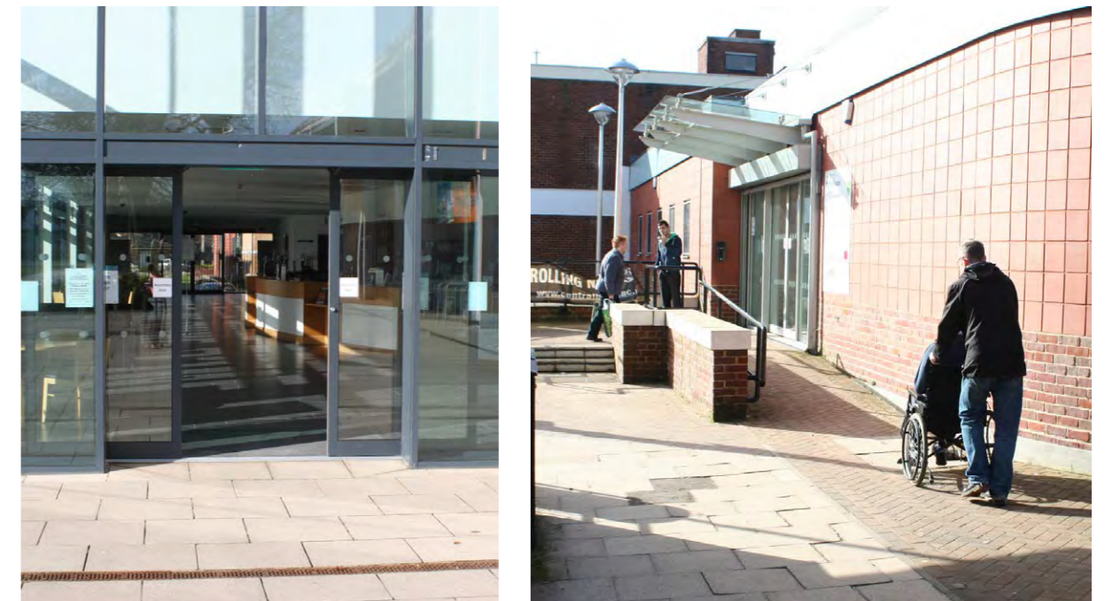
Figure 274: (left) Accessible entrance to Grove Theatre Dunstable, part of a Mixed- Use Development Figure 275: (right) Accessible Entrance to Houghton Regis Hub, Bedford Square
